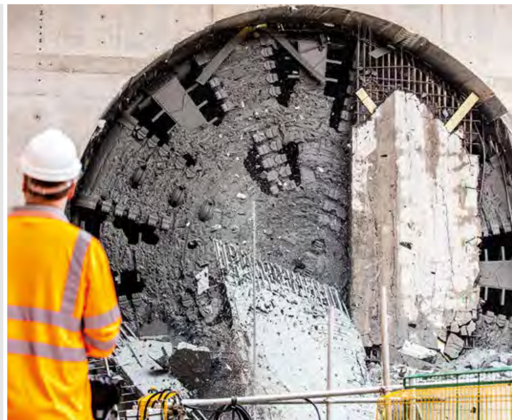
Above: Tunnel Boring Machine on the HS2 route
